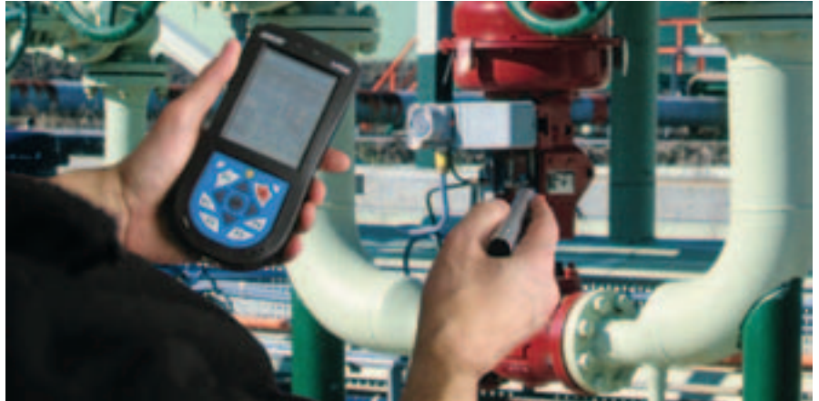
Reading the maintenance history of a pump via an embedded tag in the casing.
